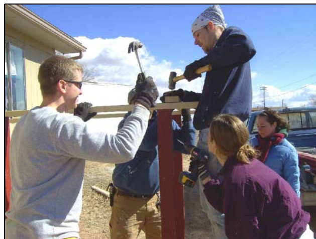
Marian University building a ramp for the handicapped
